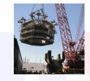
Graycor Industrial recently completed a fast-track rebuild of Blast Furnace "C" at Severstal's Dearborn, MI, plant. This complex design/build challenge required six months of preplanning to develop a unique and innovative approach to complete the construction phase within the scheduled 100-day outage.
